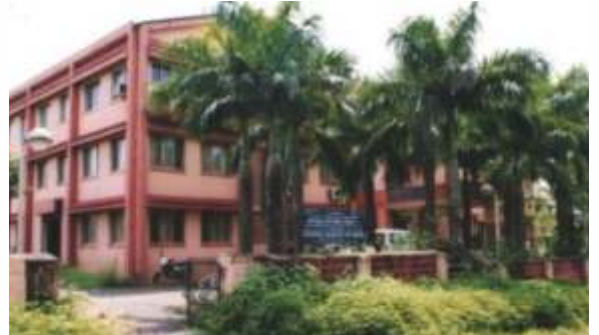
Mormugao Base Opp. Microwave Towers, Mormugao – 403 803
